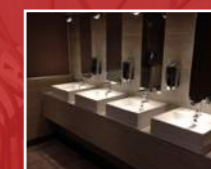
Wet Areas Waterproofing
